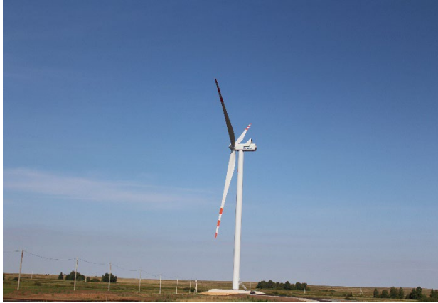
Figure 4. Burnoye Solar SPP - 100 MW and Astana EXPO-2017 WPP - 100 MW.
