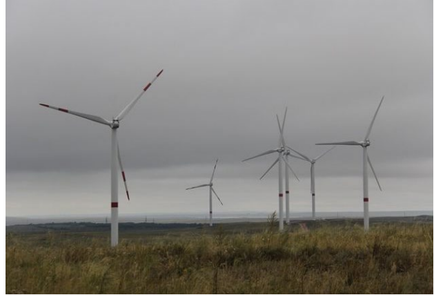
Figure 5. Saran SPP - 100 MW and Yereimentau WPP - 45 MW.
